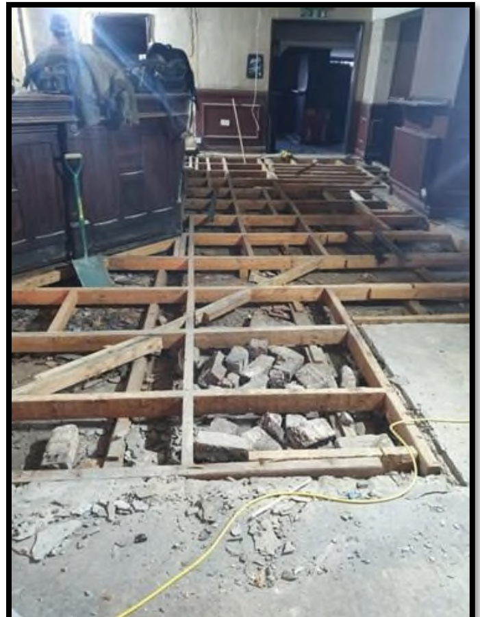
3. Structural works during refurbishment
